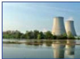
Ring monitoring for nuclear facilities
