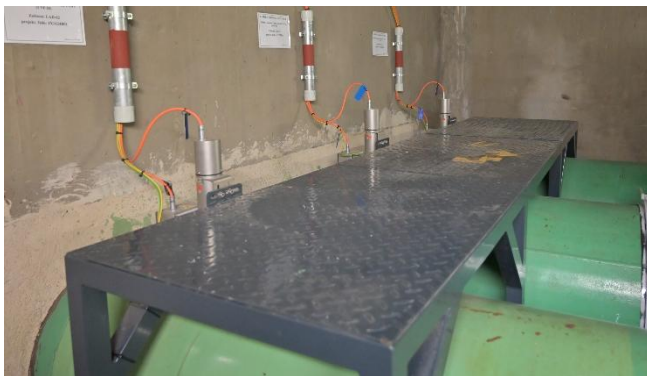
Detector installation next to the measured pipeline
